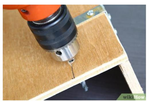
**Prill the holes for mounting.** Using the markings the board got from the sharp object you used to poke the bag as a guide.
