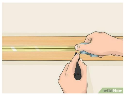
**Create 2 boards out of the 2 by 6 in (5.1 by 15.2 cm) piece to match your measurement.** Take your 2 by 6 in (5.1 by 15.2 cm) board and mark off your first cut based on the measurement between the 2 by 4 in (5.1 by 10.2 cm) boards on the ground. Cut this board the same way you cut the first set. Repeat this process again to create 2 boards of equal size.[14]
