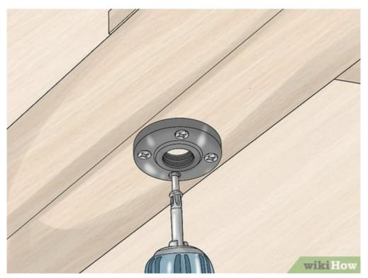
**7** Install the bracket in a ceiling joist for a hanging work stand. If you want to install the bracket in the ceiling, make sure that you either find a stud in the ceiling with a stud finder or hang it in the garage or basement on an exposed joist. Hold the bracket over the joist and use  $3^{1/2}$  in (8.9 cm) wood screws to drill it into the ceiling. Then, screw the empty end of the long pipe into the bracket by turning it clockwise until it won't turn any further.[8]
